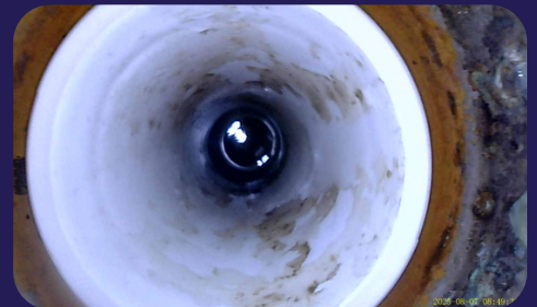
Sink after, 3 rd floor in Caldecote building
